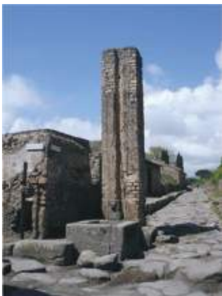
FIGURA 13 » Terminal secondary castellum aquae with turrus aquae function in Pompeii .
