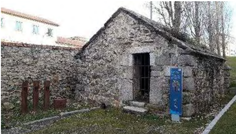
FIGURA 12 » First castellum aquae for decantation of the aqueduct in Segovia, known as La Casa de la Piedra. Source: Francisco Javier Espejo.
